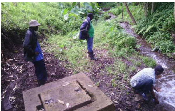
Farmers and staff repairing drainage in the farms
