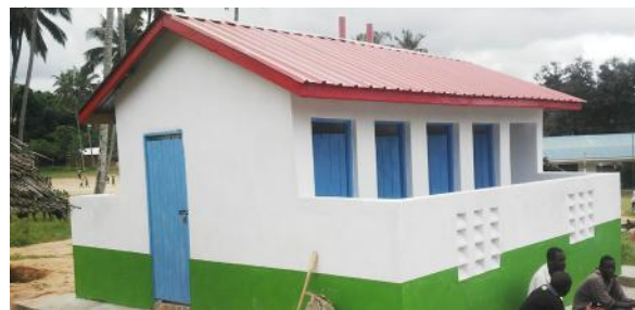
TPC built a toilet block for Tsakorolov Primary School
