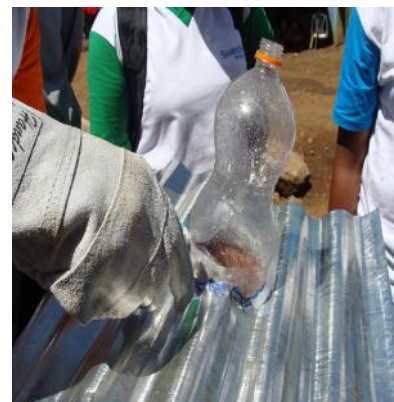
Making of the daylights
