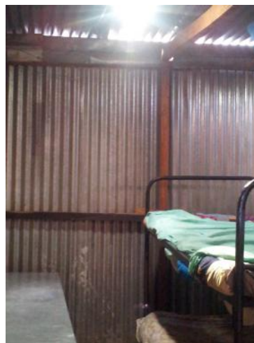
After daylights were installed
